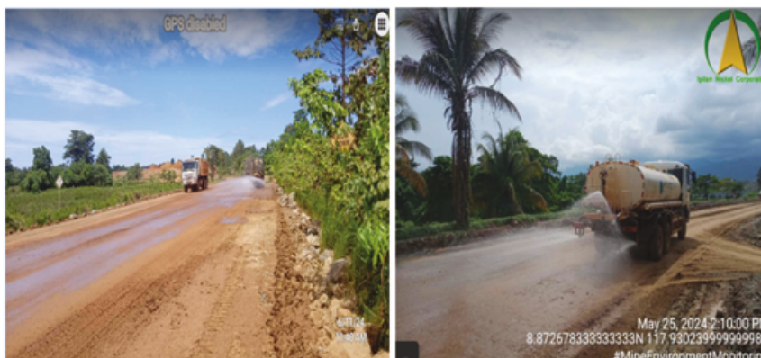
Figure Nos. 1 & 2: Road Watering
